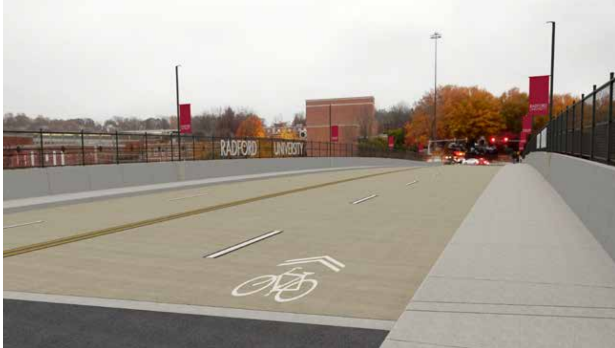
University Drive Bridge Update
