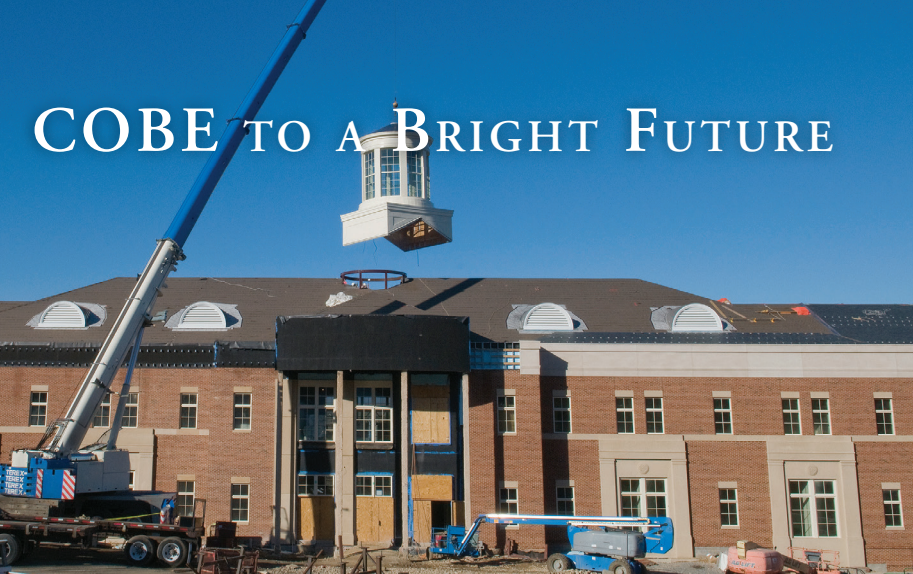
WEIGHING MORE THAN SEVEN TONS, IS PLACED ATOP THE NEW COBE BUILDING.
